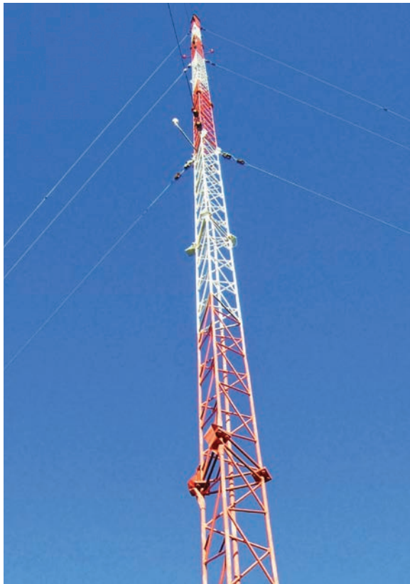
FIGURE 2.22 Monopole antenna
