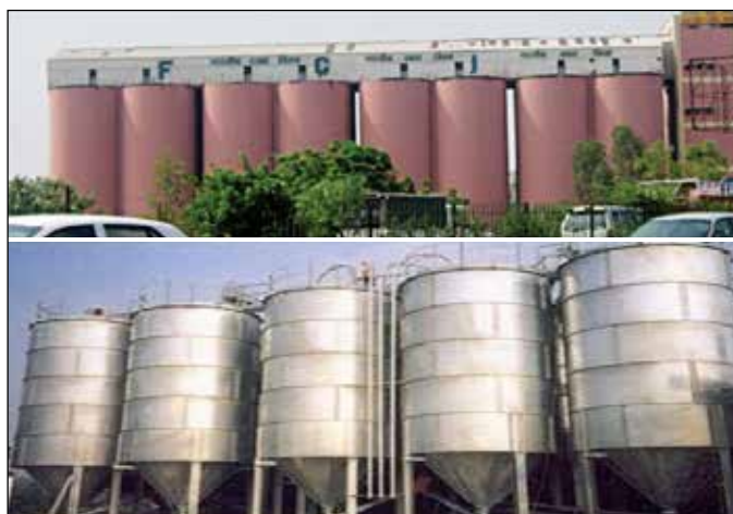
Fig. 3: Concrete silos at FCI, Mayapuri, New Delhi, and Commercial hopper bottom storage silos
