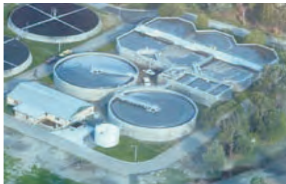
Figure 10.7 An aerial view of a sewage plant
