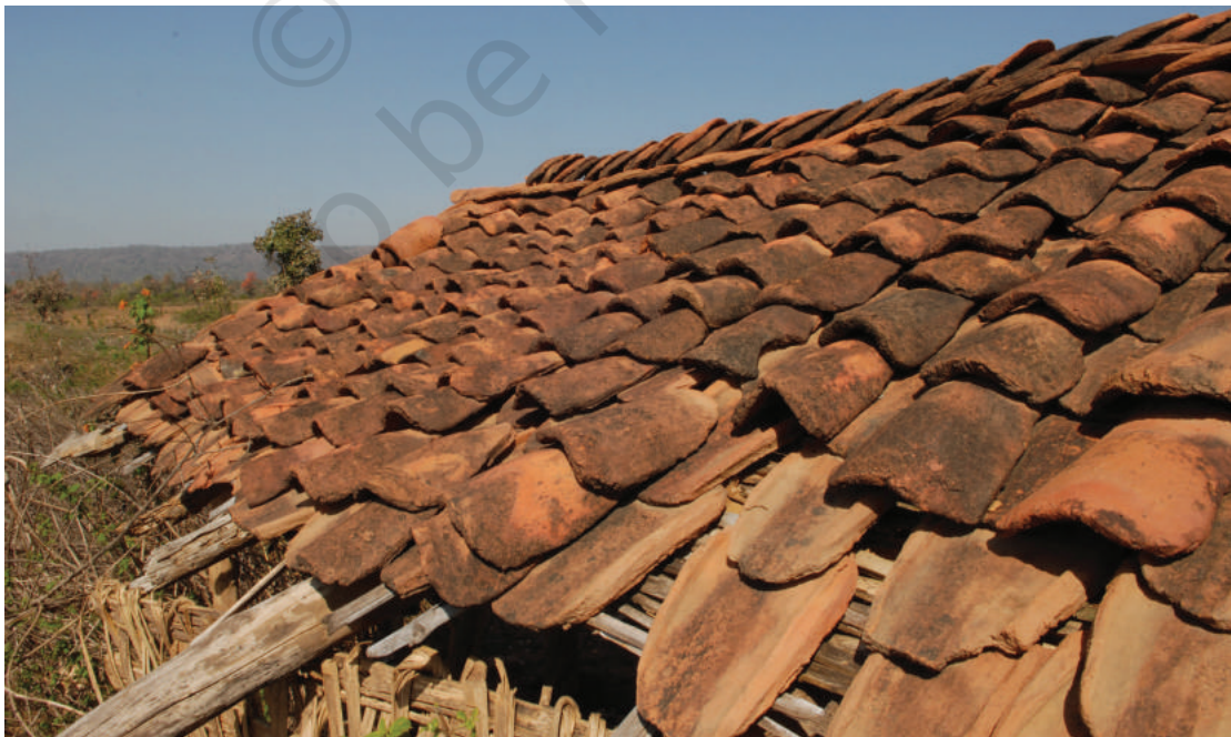
Clay roof-tiles, Madhya Pradesh
