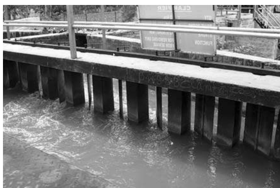
Fig. 18.4 Grit and sand removal tank
