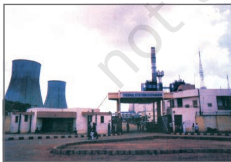
Fig 3.10: A view of a Thermal Power Station
