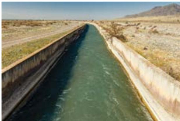
One such canal shown above is of width 5.4 m wide and depth 1.8 m deep through which water is flowing with a speed of 25 km/hour.
