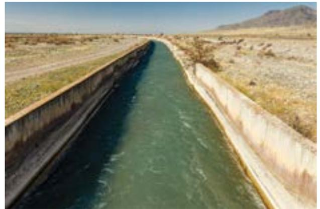
One such canal shown above is of width 5.4 m wide and depth 1.8 m deep through which water is flowing with a speed of 25 km/hour.
