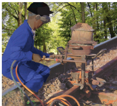
Figure 3.11 Thermit process for joining railway tracks
