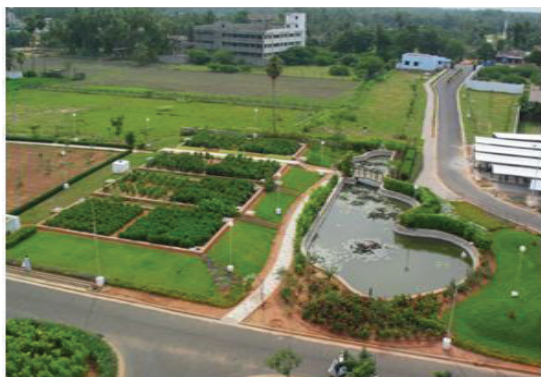
Fig .12.7 (a) DEWATS system at Auroville
