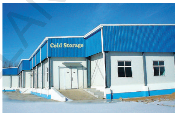
Fig-28 Cold storage unit
