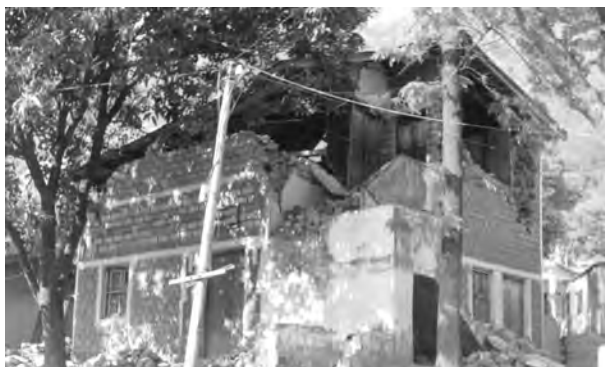
Figure 7.1 : A Damaged Building Due to an Earthquake
