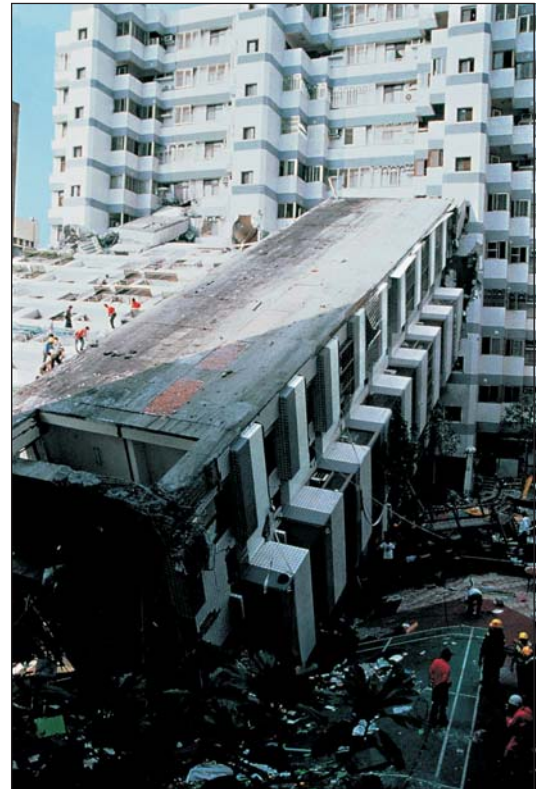
The building has tilted as a result of column failure & has partly damaged the nearby building (Taiwan 1999). (By Bachmann H., Sesimic Conceptual Design of Buildings)
