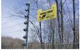
Fig. 6 Electrified Fence
