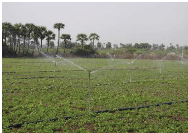
Fig. 15.6 Sprinkler Irrigation System
