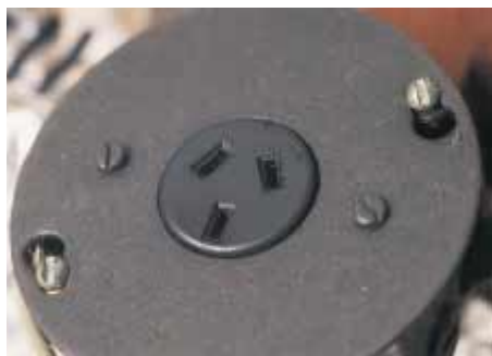
Figure 28.29 A power connection for a 240-V appliance.
