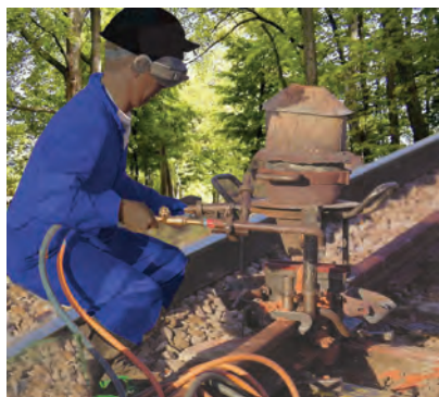
Figure 3.11 Thermit process for joining railway tracks
