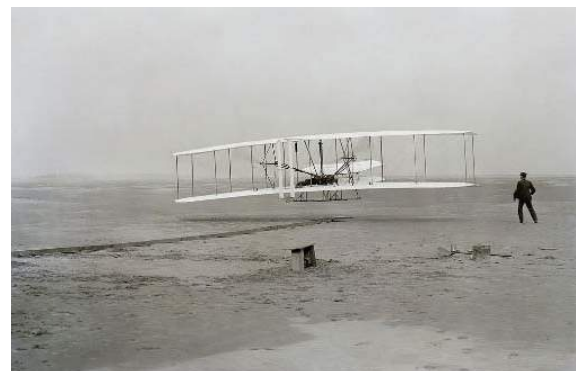
First successful flight of the Wright Flyer, by the Wright brothers. The machine traveled 120 ft (36.6 m) in 12 seconds at 10:35 a.m. at Kill Devil Hills, North Carolina. Orville Wright was at the controls of the machine, lying prone on the lower wing with his hips in the cradle which operated the wing-warping mechanism. Wilbur Wright ran alongside to balance the machine, and just released his hold
