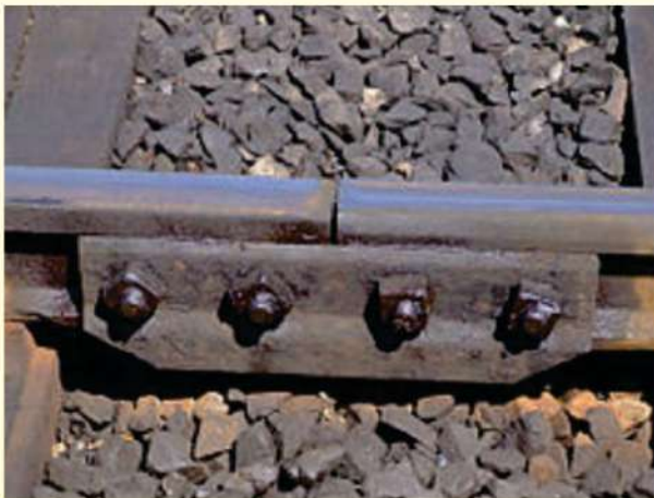
Fig 4.14 Fishplate bolted joint
