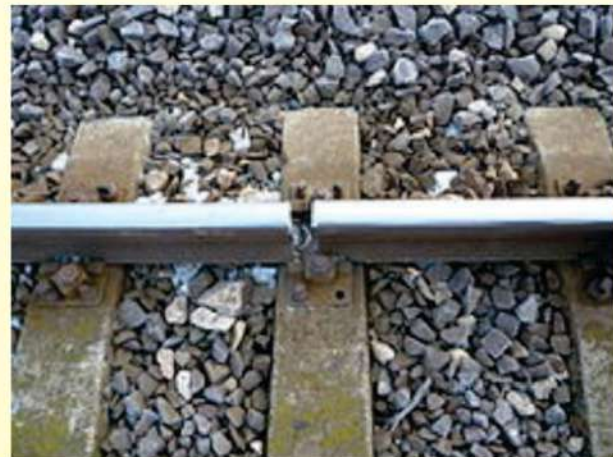
Fig 4.15 A rail break
