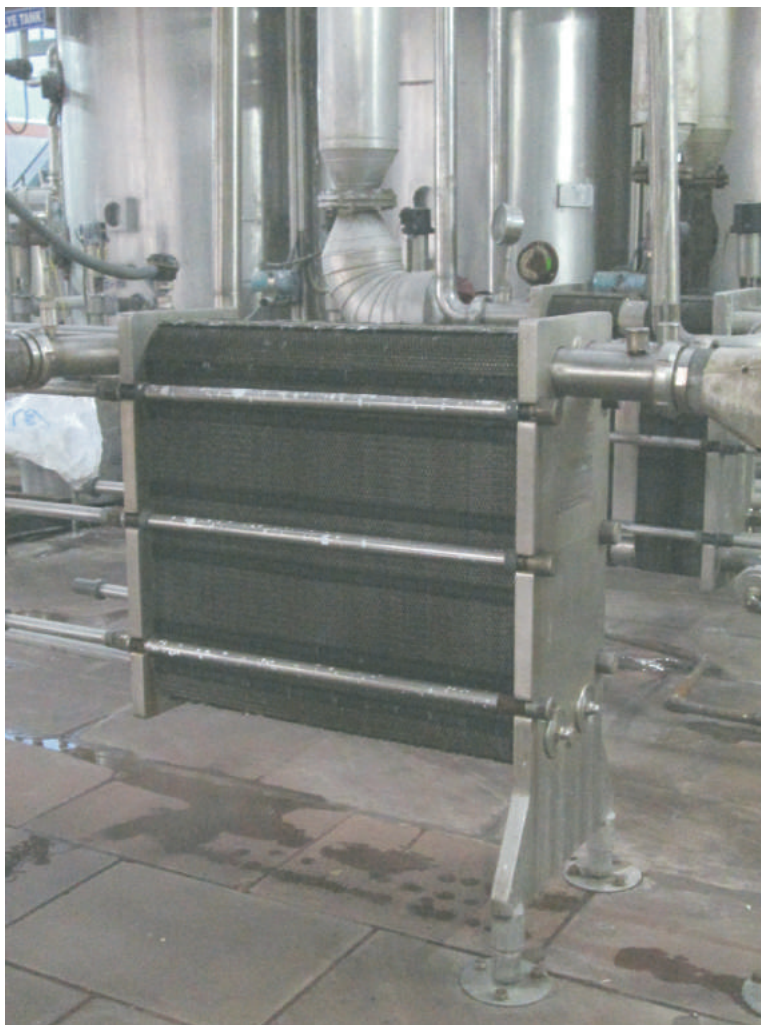
Fig.7.1. Plate heat exchanger
