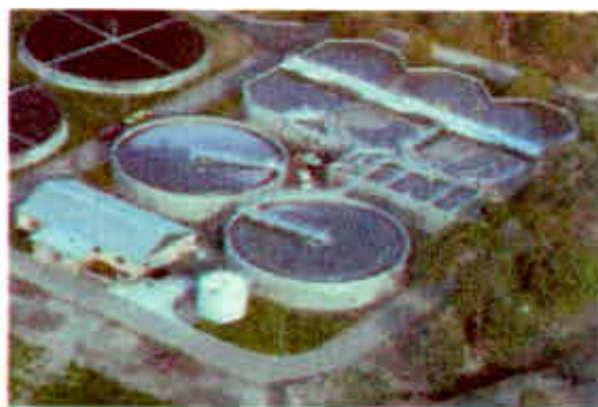
Figure 10.7 An aerial view of a sewage plant
