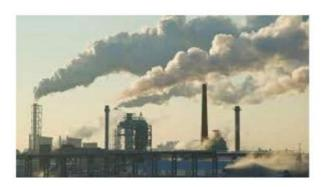
\* Tip: The chimneys in the factories are made long. The long chimney carries the harmful smoke and gases away from the ground and reduces the harmful effects of these gases.
