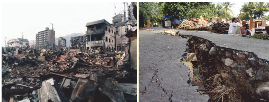
Fig. 30.3 Collapsing of buildings and build up debris
