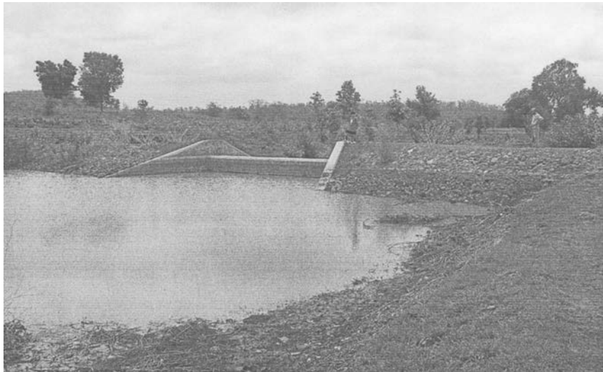
A small dam
