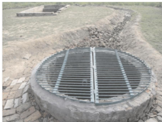
Groundwater recharge through abandoned well
