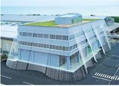
It is the building which is designed by the Japan which is strong enough to face the wild earthquake. The strings are being attached by the fibre.
