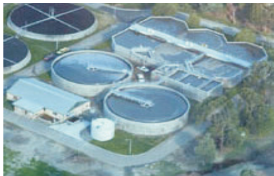
Figure 10.7 An aerial view of a sewage plant
