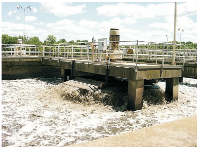
Figure 10.6 Secondary treatment
