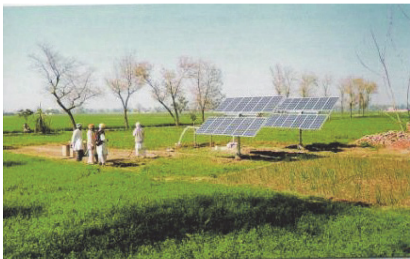
Fig. 12.2 Photovoltaic Water Pumping
