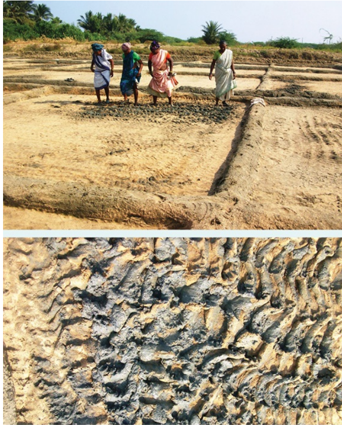
Fig 4.13, 4.14 Salt pan leveling work known as 'Adugetha', which makes the pan impervious
