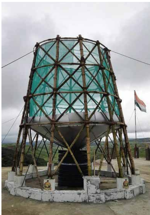
Bamboo Water Tower, traditional method of water preservation and storage
