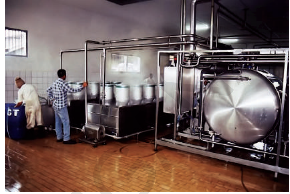
Fig-7 Chilling center
