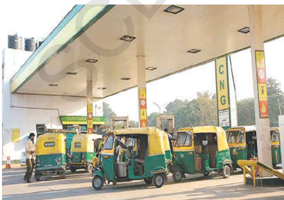
Fig - 3: CNG gas filling station
