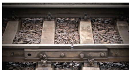
Figure 7.1 Gap in railway track
