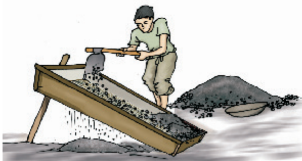
Fig 5.7 Pebbles and stones are removed from sand by sieving
