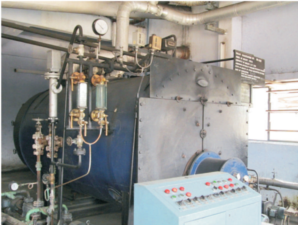
Fig.12.1. Oil fired boiler
