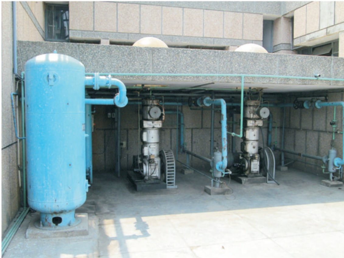
Fig.12.7. Equipment for producing compressed air
