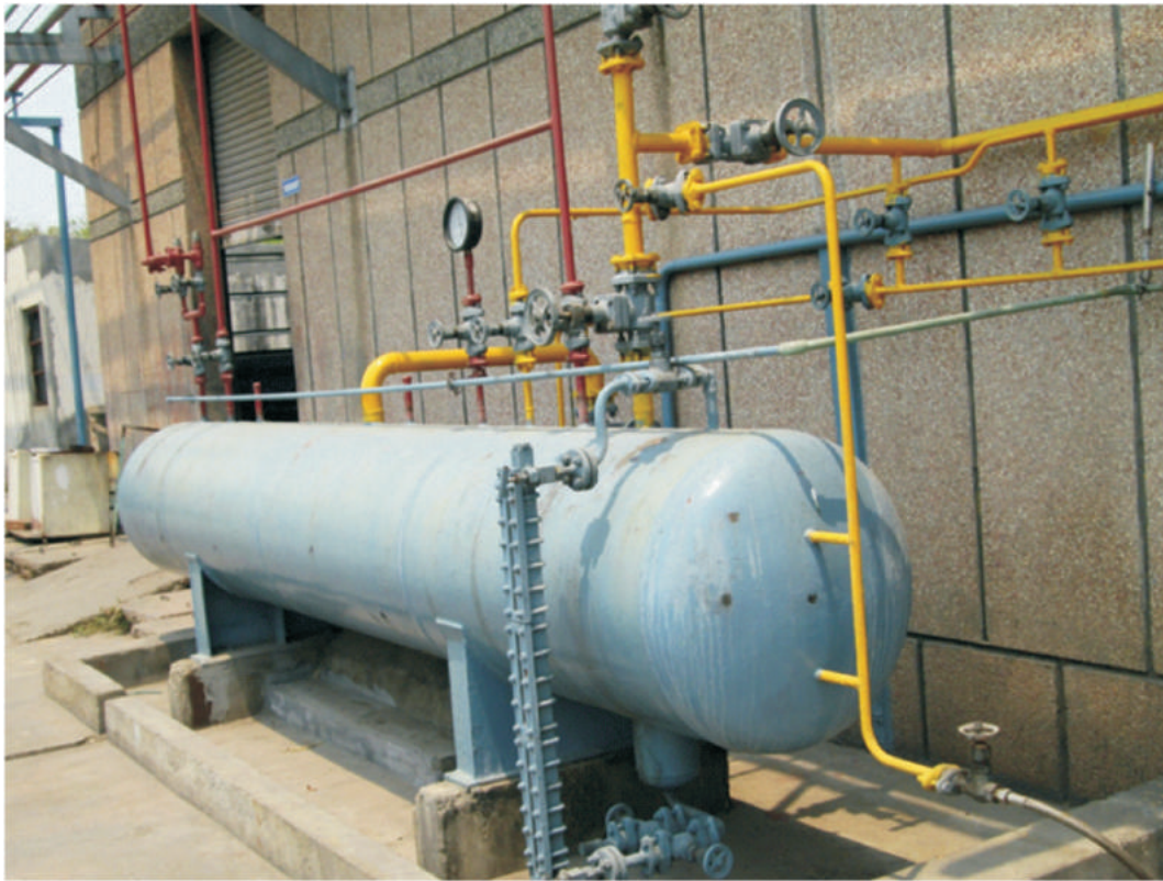
Fig.12.4. Ammonia reservoir/tank for the refrigeration system
