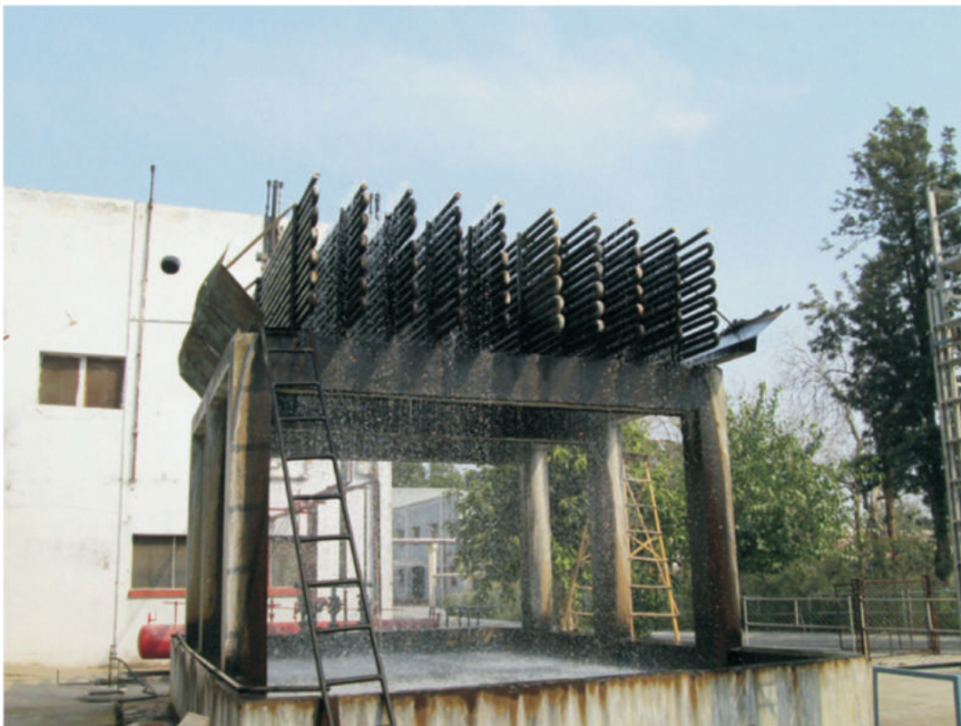
Fig.12.5. Water cooled condensor
