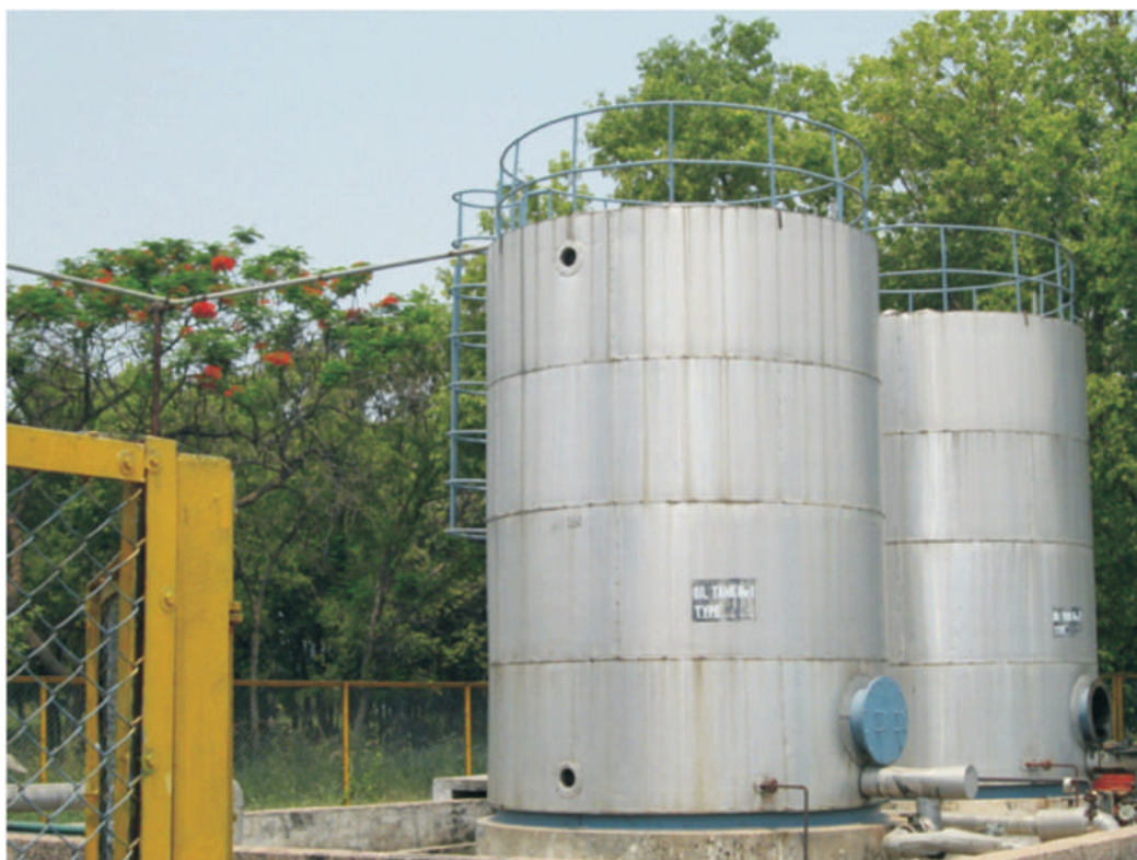
Fig.12.2. Oil tanks for boiler
