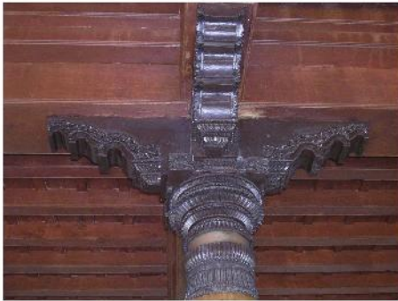
Detail of an ornate pillar in a landlord's house, Chettinad, Tamil Nadu
