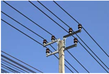
Fig. 1.5 Concrete pole
