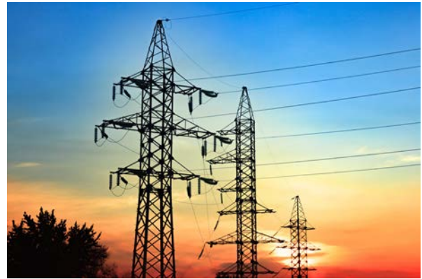
Fig. 1.7 Latticed steel tower
