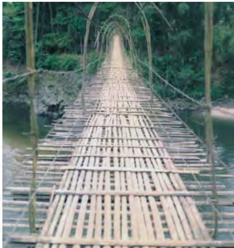
Cane-and-bamboo suspension bridge over a torrential river in Along, Arunachal Pradesh
