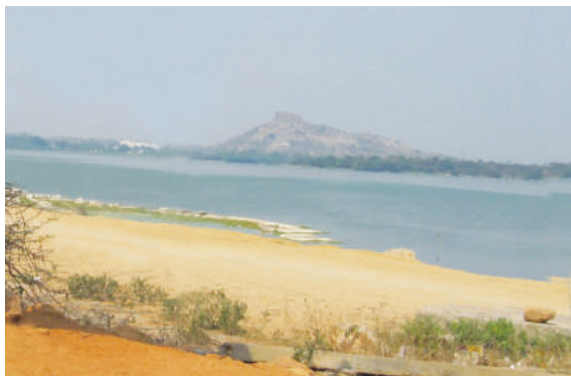
fig-8: Edulabad Water Reservoir
